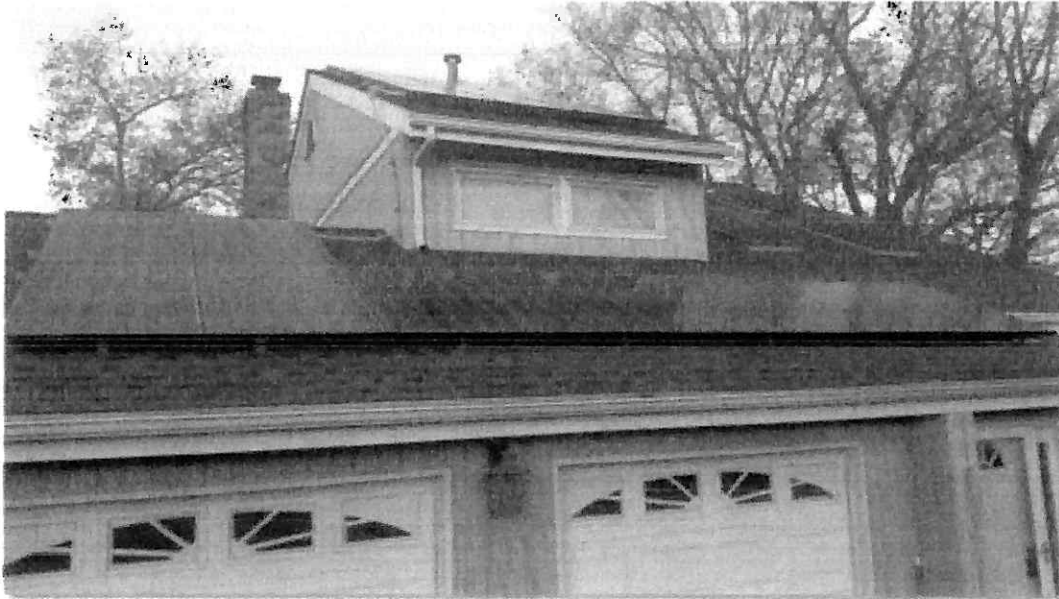
Figure 1: Solar panels installed on a house w/ black frames and black mounting system.
